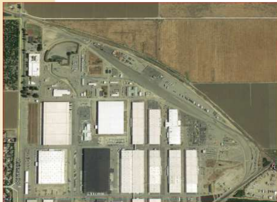
After - See left and center of the photograph where four warehouses were demolished, and three new warehouses, and an office building were constructed.
